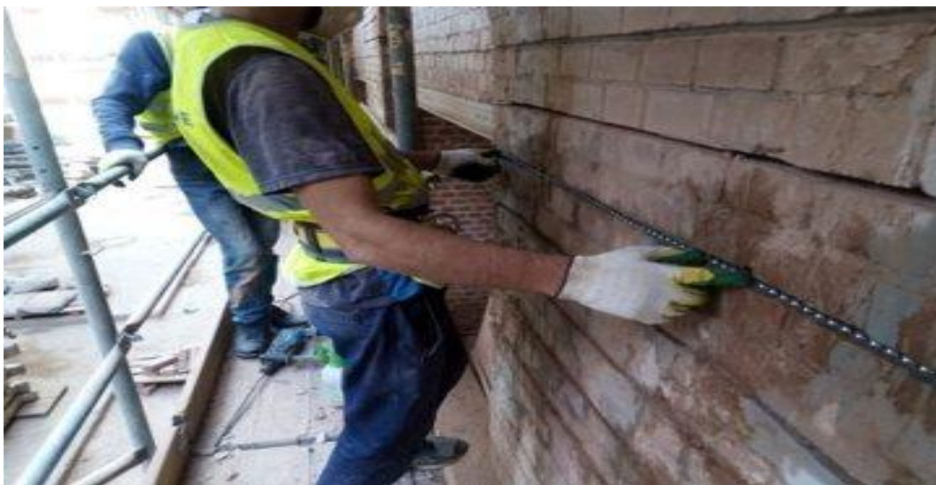
3.4-rasm.RSA spiral anker bilan mustahkamlash ishlari
